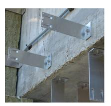
VFM is a Magnelis steel carrier system designed for use as either a standard helping hand style system, or more commonly a floor spanning carrier system. It has a much higher melting point than a standard aluminium systems; 1425-1540 C vs 660 C
