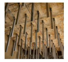
The VitraFix® Soffit System (VFS) offers a customizable solution for your soffit needs. The drop can be adjusted to meet your specific requirements and the system is composed of brackets made from either 5251/H22 or 6063/T6 grade aluminium.
