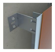
VF1 system uses helping brackets installed against the wall and then aluminium profiles.
