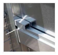
VF4 system uses horizontal Channel rails and brackets and uses the VF1 or VF2 subframe systems similar to the VF3 system however the brackets are attached to aluminium panels either by stud welding or structurally bonding.
