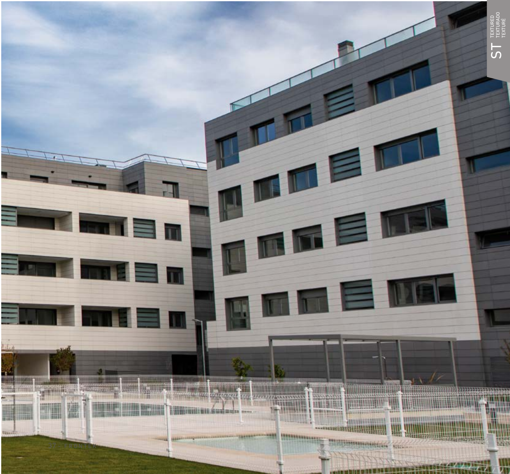
SPAIN - CASTILLA-LA MANCHA RESIDENTIAL BUILDINGS ST5006 ● JÚPITER ●
