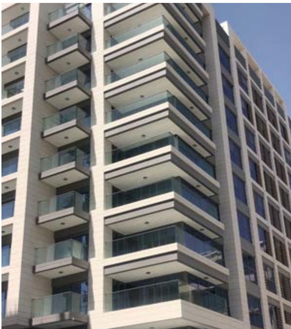
DHAFRA PROJECT - ABU DHABI RESIDENTIAL BUILDING
