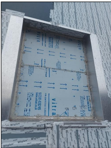
Photograph No. 12 - Window interface external
