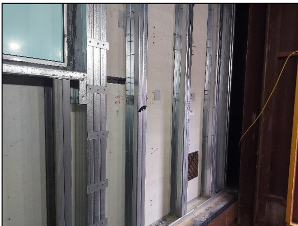
Photograph No. 10 - Lower level SFS
