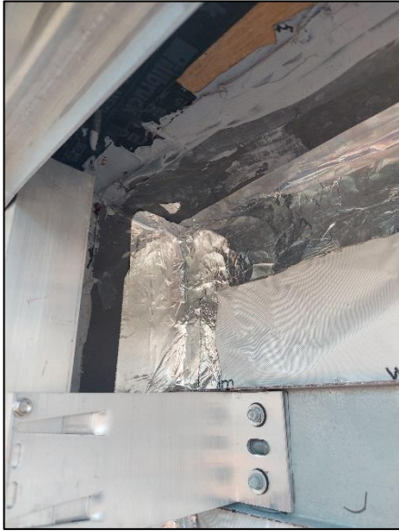
Photograph No. 22 - Perimeter detail to UL Steelwork
