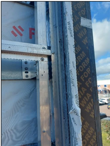
Photograph No. 25 - Edge of sample with panels removed
