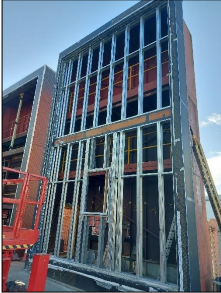
Photograph No. 32 - Showing SFS with sheathing boards removed
