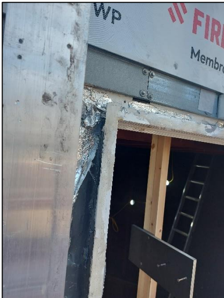
Photograph No. 29 - Window interface
