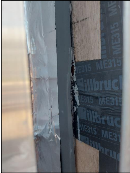
Photograph No. 28 - Perimeter detail to UL Steelwork
