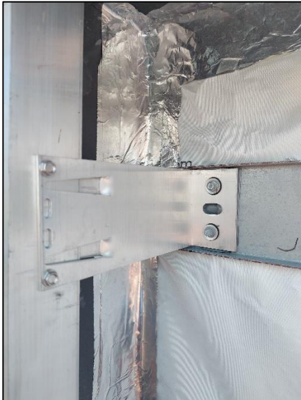
Photograph No. 23 - Bracket
