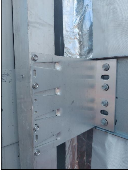
Photograph No. 24 - Double bracket
