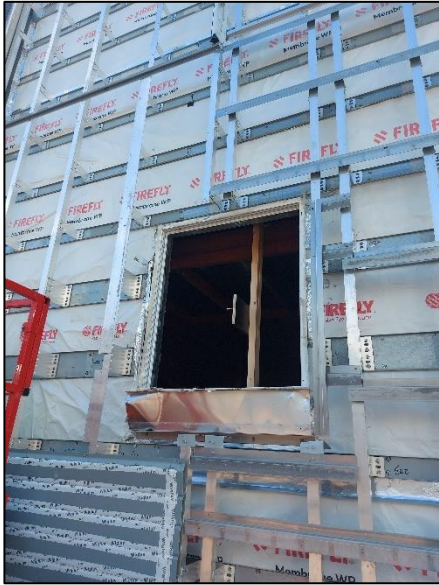
Photograph No. 18 - Window Pod Removed
