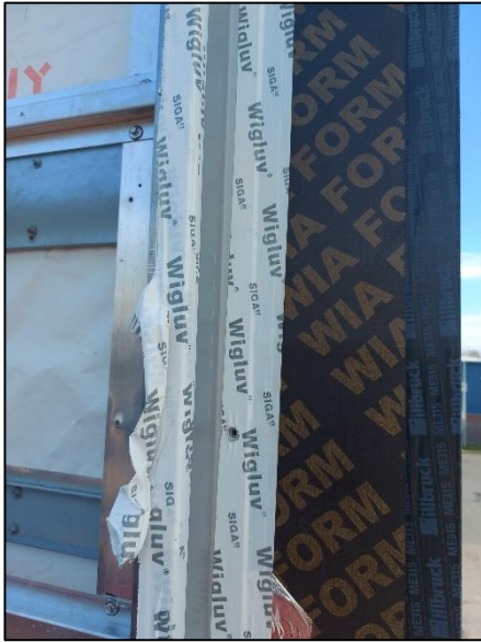
Photograph No. 26 - Perimeter flashing top section
