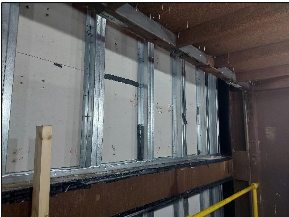
Photograph No. 13 - Upper Level SFS
