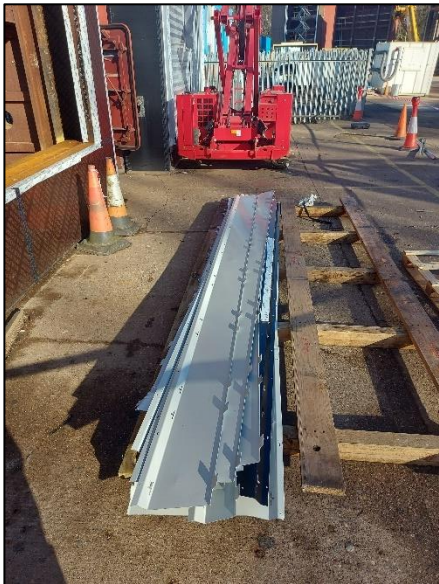
Photograph No. 17 - Panels removed
