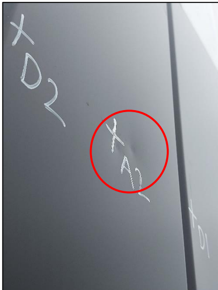
Photograph No. 6 – Damage caused following impact ref A2
