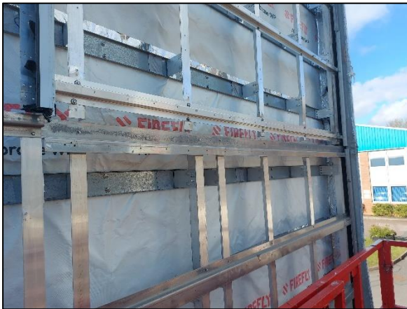
Photograph No. 27 - Connection between bottom and top half of panels
