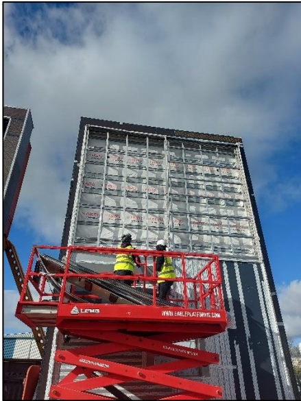
Photograph No. 16 - Top half of panels removed
