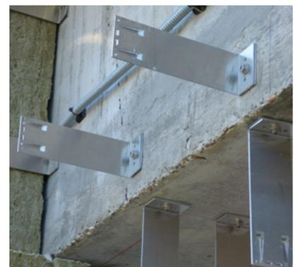
VFM is a Magnelis steel carrier system designed for use as either a standard helping hand style system, or more commonly a floor spanning carrier system. It has a much higher melting point than a standard aluminium systems; 1425-1540 C vs 660 C
